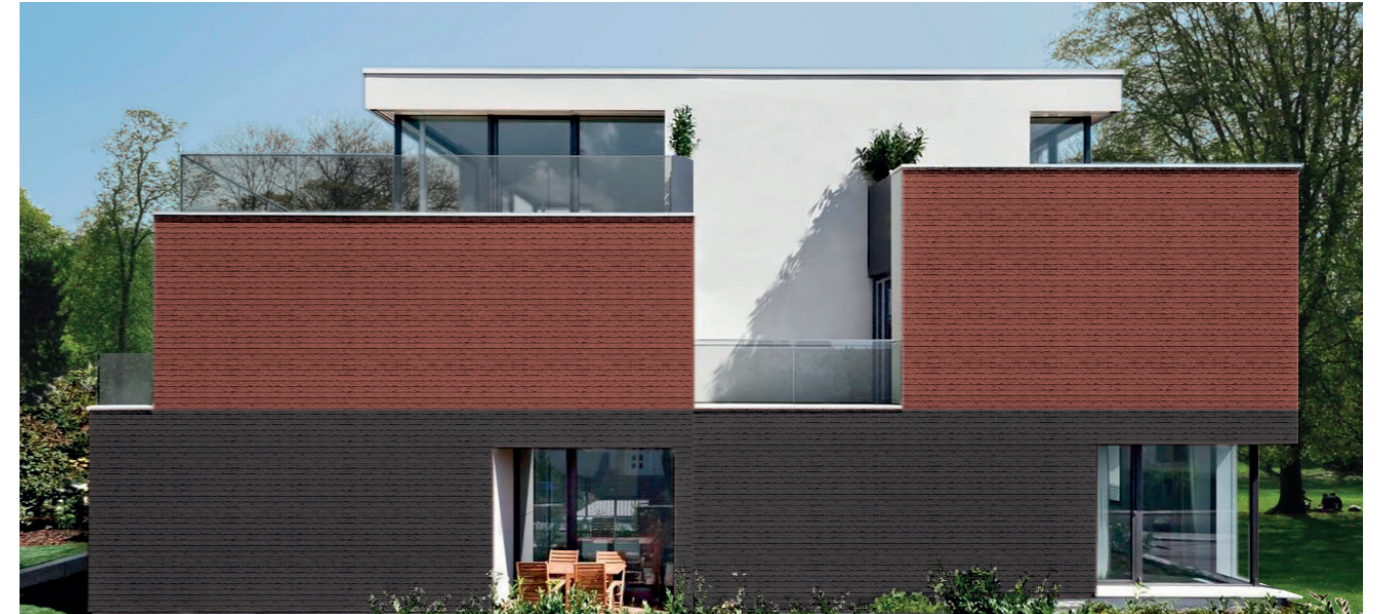
Structure 2 - Weber Strate
